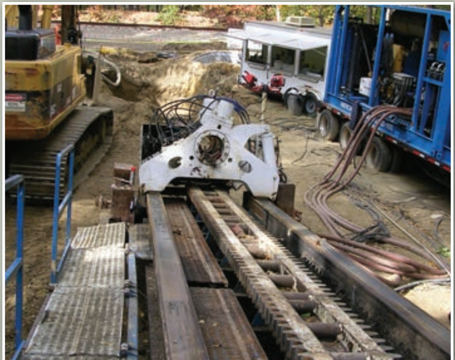
Pipe ramming the 42-in. steel sleeve under the railroad.
