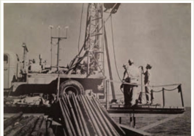
Figure 2. Drilling soil borings off moored barge in 1957.
