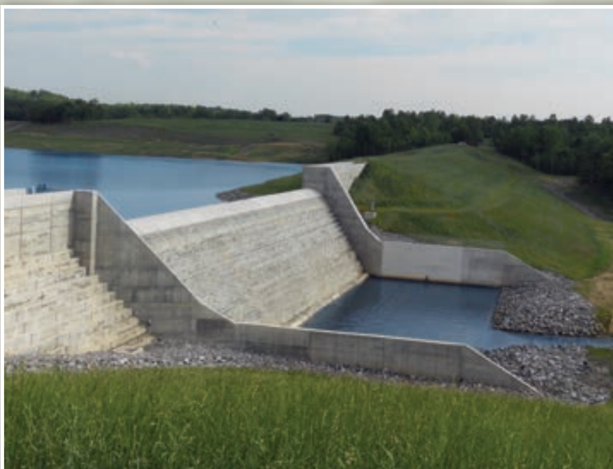
Completed Deep Creek Watershed 5D Dam.
