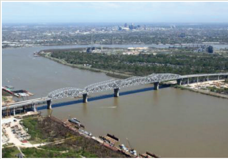
The Huey P. Long Bridge, New Orleans (Photo Credit: Louisiana TIMED project photo album)
