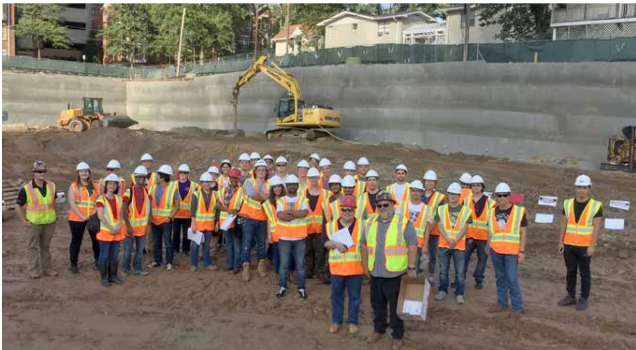
2015 ground modification fieldtrip to Juniper Street in Atlanta, GA; Paul Mayne and John Wolosick in front of group.
